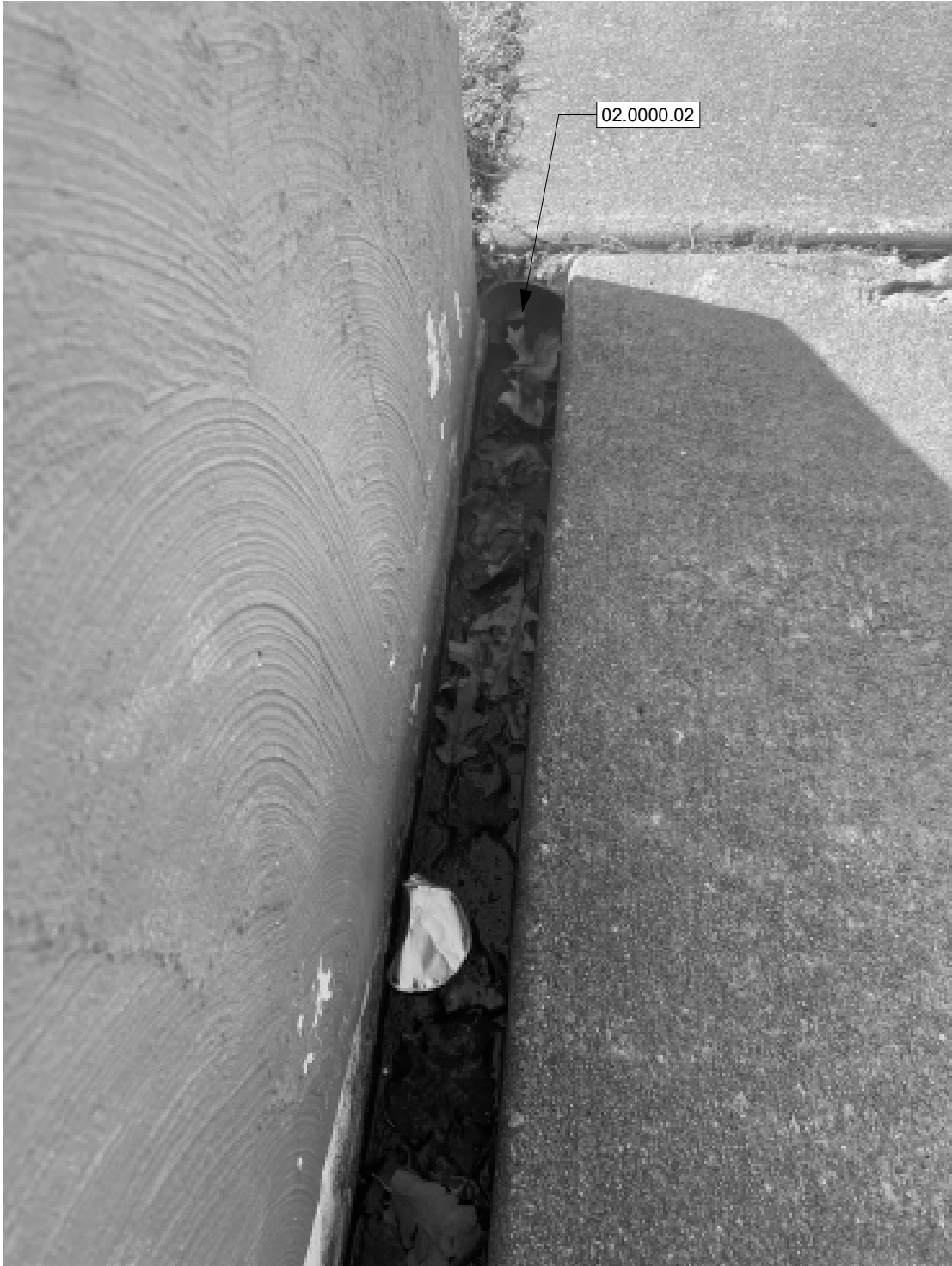
TUNNEL GUTTER CHANNEL AT SOUTH ENTRANCE
