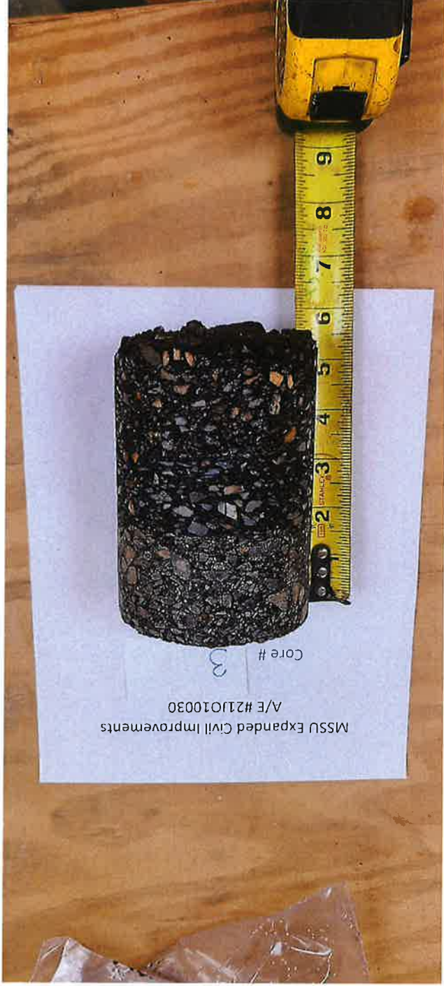
21J010030 MSSU Expanded Civil Improvements
