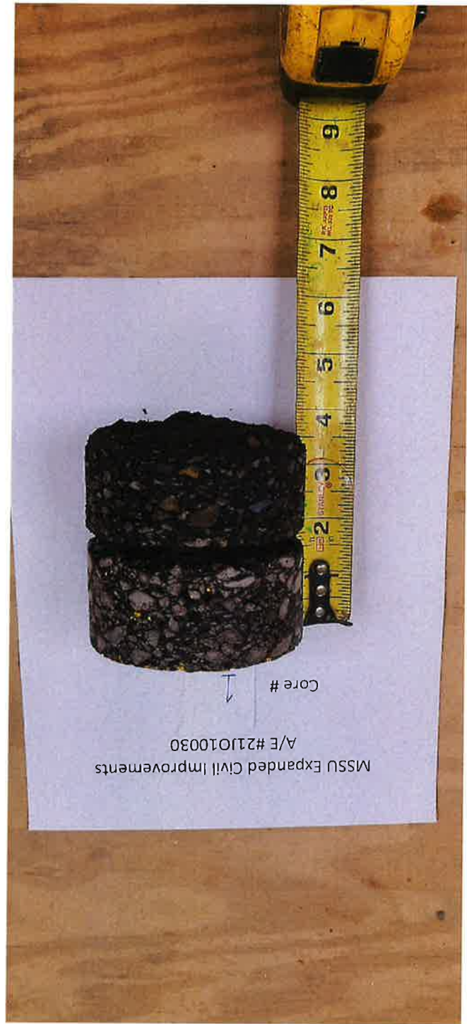
21J010030 MSSU Expanded Civil Improvements
