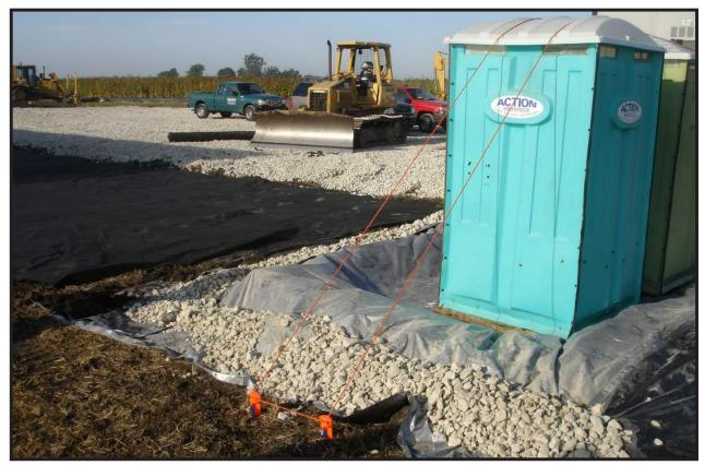
Figure 6.18 Typical port-a-potty with secondary containment and tie downs. Source: BFA Inc.
