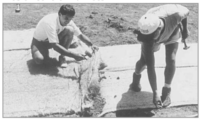
Figure 6.30 Follow manufacturer's recommendations to successfully install erosion control blankets or matting. The manufacturer of this high velocity blanket called for stapling every two feet and a check slot wherever two sections were joined. This blanket was used to protect soil and establish grass in a waterway on the August Busch Memorial Conservation Area
