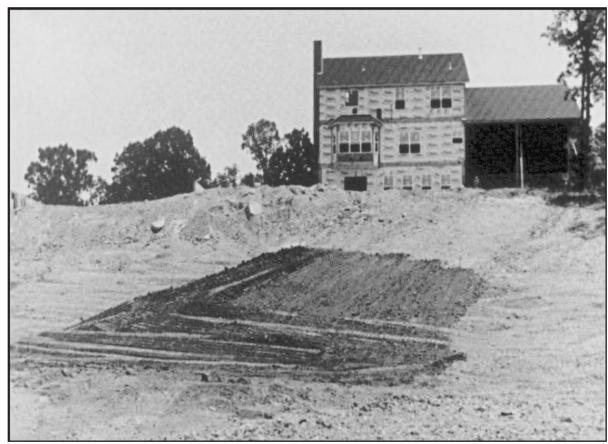
Figure 6.16 It's important to mix or incorporate topsoil with the underlying subsoil to prevent sloughing on sloping soils. Source: *C. Rahm, NRCS. St. Louis Co.*
