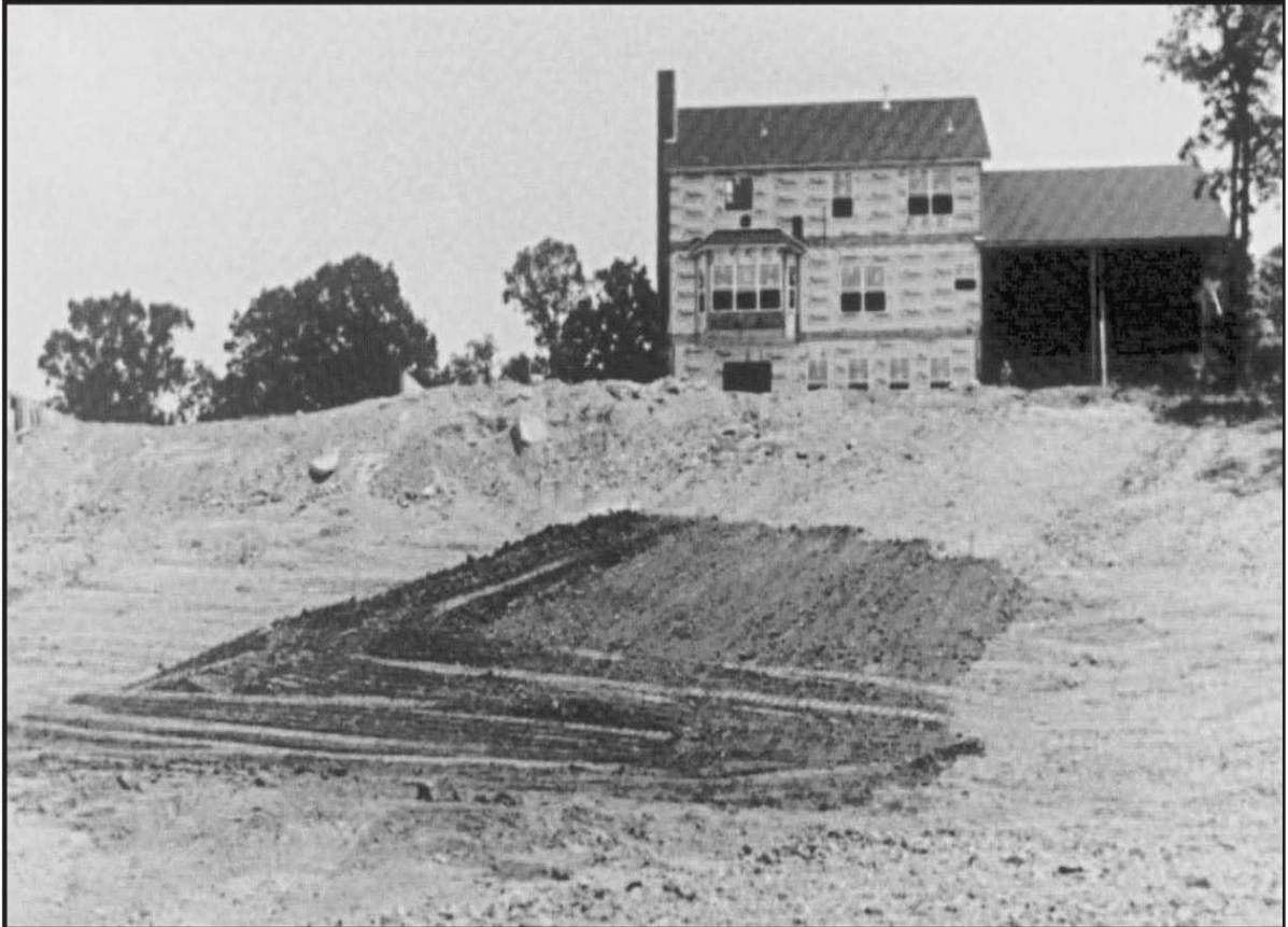
Figure 6.16 It's important to mix or incorporate topsoil with the underlying subsoil to prevent sloughing on sloping soils.
