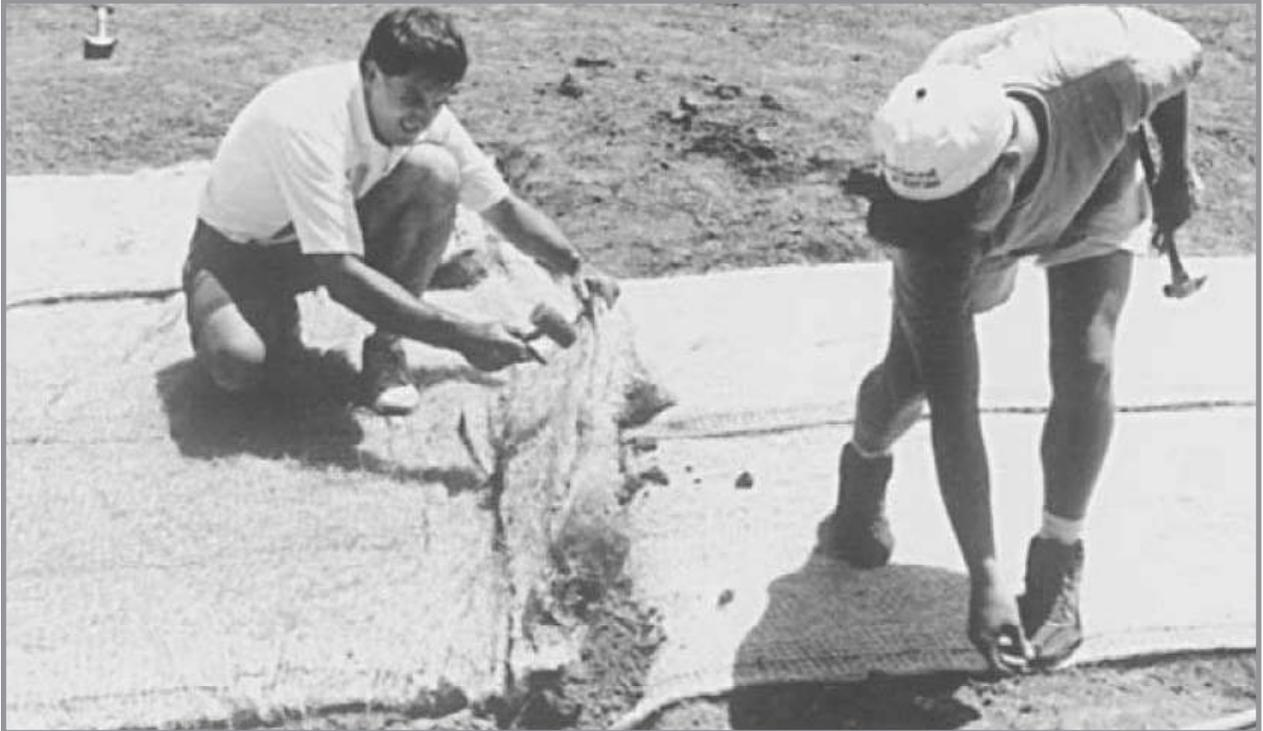
Figure 6.30 Follow manufacturer's recommendations to successfully install erosion control blankets or matting. The manufacturer of this high velocity blanket called for stapling every two feet and a check slot wherever two sections were joined. This blanket was used to protect soil and establish grass in a waterway on the August Busch Memorial Conservation Area
