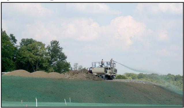
Figure 6.26: Hydroseeding over matt armoring on a steep slope to promote vegetation growth and prevent erosion. Source: Florida Erosion and Sediment Control Designer and Reviewer Manual, June 2007
