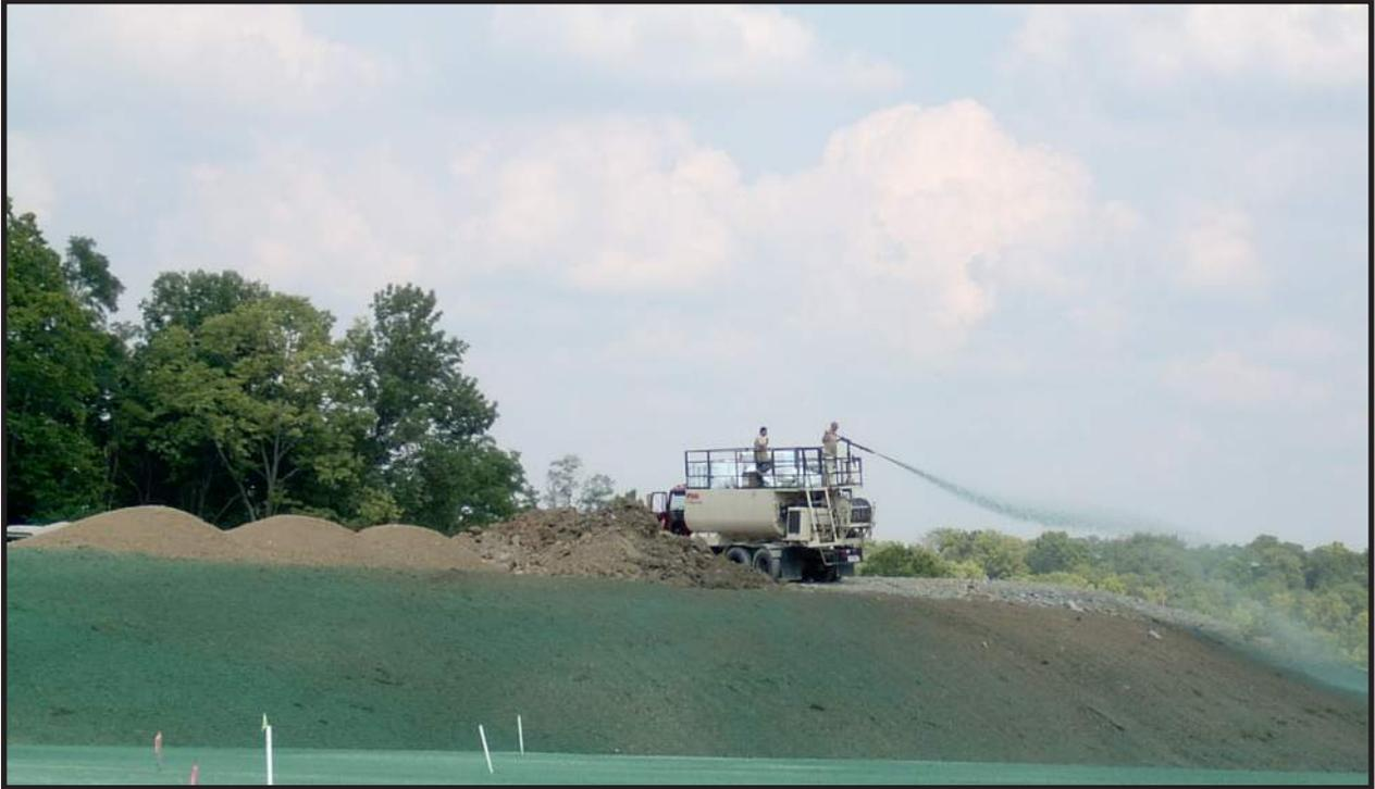
Figure 6.26: Hydroseeding over matt armoring on a steep slope to promote vegetation growth and prevent erosion.
