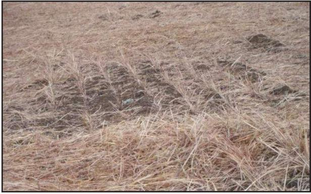
Figure 6.28 Crimped straw. Source: ABCs of BMPs, LLC.
